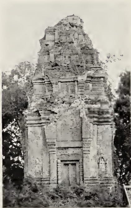
326. Brick tower, Bakong; ninth century.
